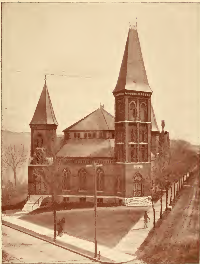
NORTH PRESBYTERIAN CHURCH, CHENANGO ST., BINGHAMTON, N. Y.
